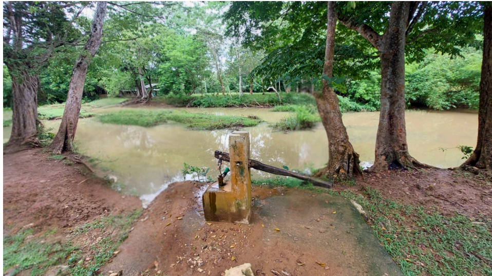
Figure 1.2. The original shallow water pump well in Sitio Padungsol, positioned next to the visibly turbid stream that served as the community's primary water source.
